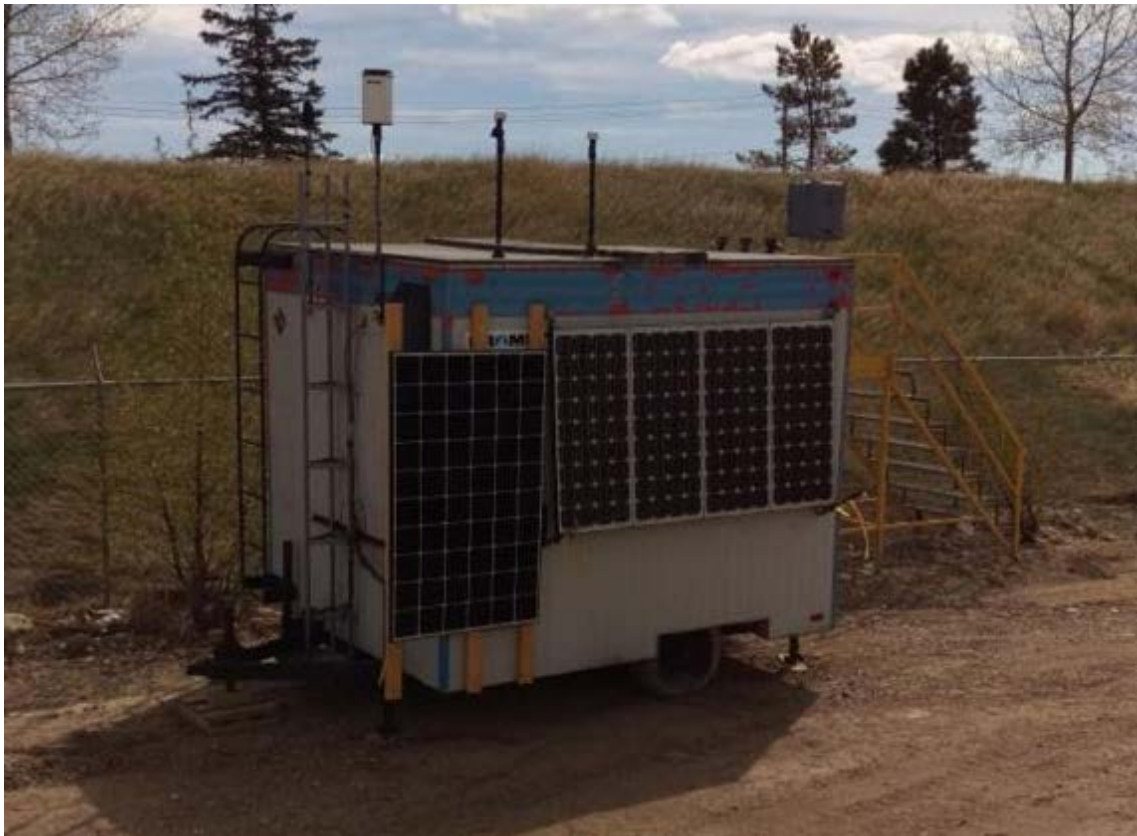
Figure A2: Picture of West Berm Station
